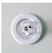
Sidewall Sprinkler
